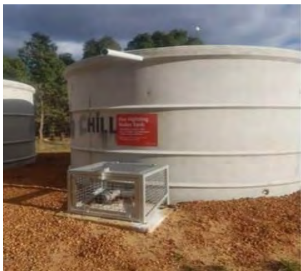
Strategic 47,000 Litre Concrete Tank & Protected Fittings
