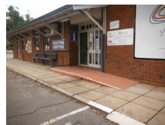
Access to CRC Building
