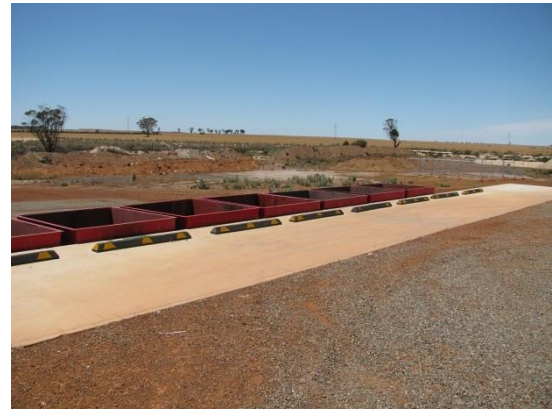
Kondinin Transfer station
