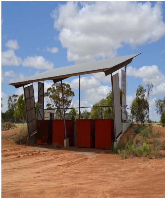
Meckering Transfer station
