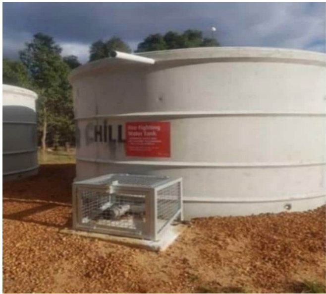
Example Strategic 47,000 Litre Concrete Tank & Protected Fittings
